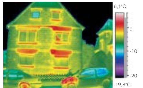
Hot spots due to bad insulation
